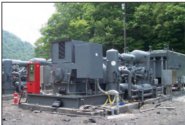
■ (Left) This Dearing Compressor and Pump Co. two-stage package includes a Caterpillar G3608 gas engine driving an Ariel JGC/4 compressor at a rated speed of 1000 rpm. (Right) Two three-stage Dearing 2250 hp (1678 kW), 900 rpm synchronous motor-driven Ariel JGC/4 compressors are shown being readied for commissioning at an Appalachian Basin customer site.
