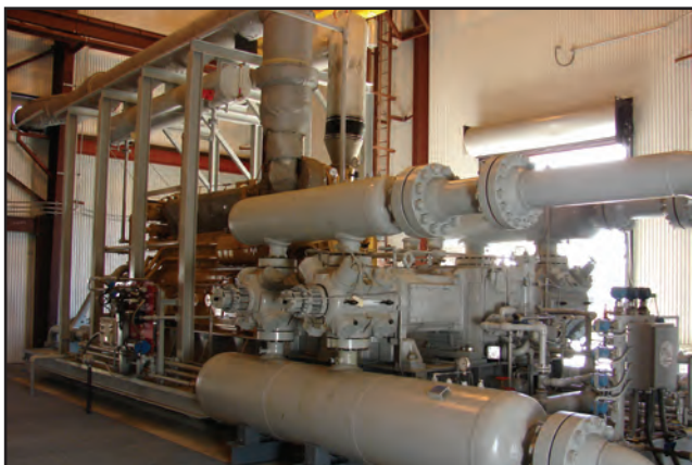
■ (Left) This Dearing Compressor and Pump Co. two-stage package includes a Caterpillar G3608 gas engine driving an Ariel JGC/4 compressor at a rated speed of 1000 rpm. (Right) Two three-stage Dearing 2250 hp (1678 kW), 900 rpm synchronous motor-driven Ariel JGC/4 compressors are shown being readied for commissioning at an Appalachian Basin customer site.
