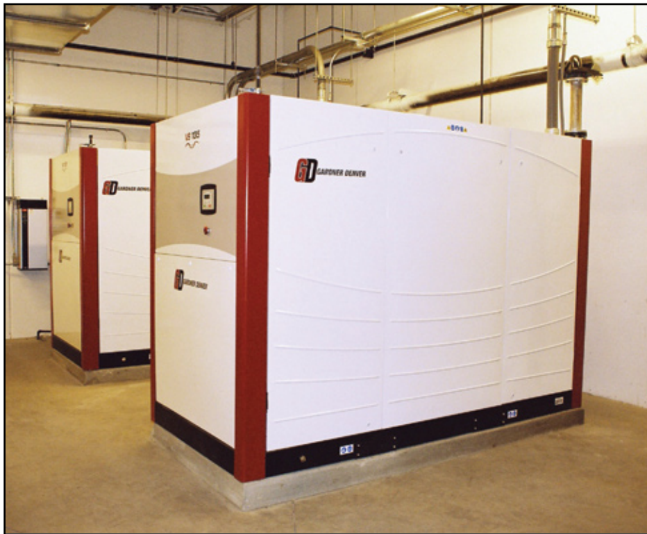
Two Gardner Denver VS135 single-stage, air-cooled, variable speed drive compressors rated at 802 CFM @ 125 PSIG. These units are being operated in a three-shift plant, 7 days per week. Estimated annual energy savings are more than $50,000.
