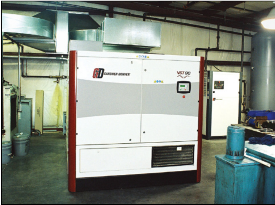
A Gardner Denver VST-90 two-stage, air-cooled, variable speed drive compressor rated at 677 CFM @ 100 psig. This unit is installed at a manufacturer of building supplies and operates a two-shift plant, 5 days per week. Estimated annual energy savings are more than $25,000.
